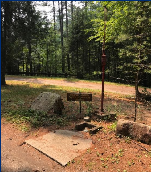
Existing Dump Station
